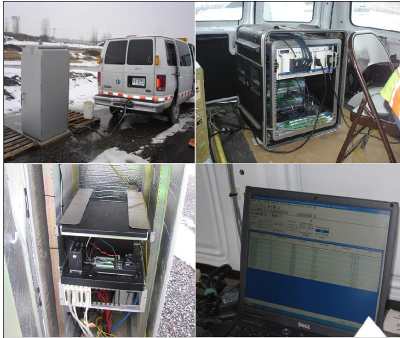
Figure 3-7. MnROAD Pavement Response Data Collection System
